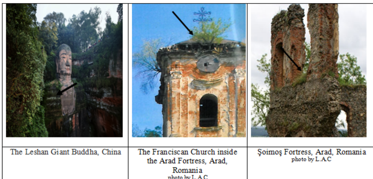
Figure 6. The “salts weathering” of the limestone material
